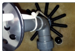
Internal union for ease of maintenance
